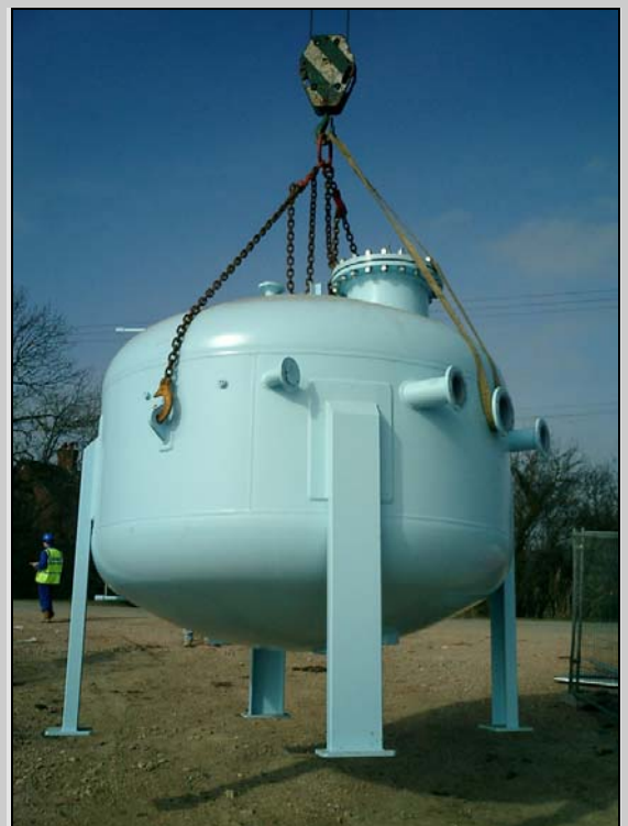
The large vacuum vessel being lifted into place
